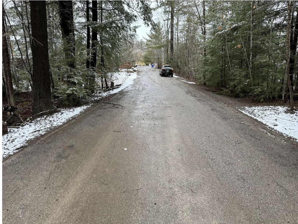
Photo 1 Entrance Roadway Overview
