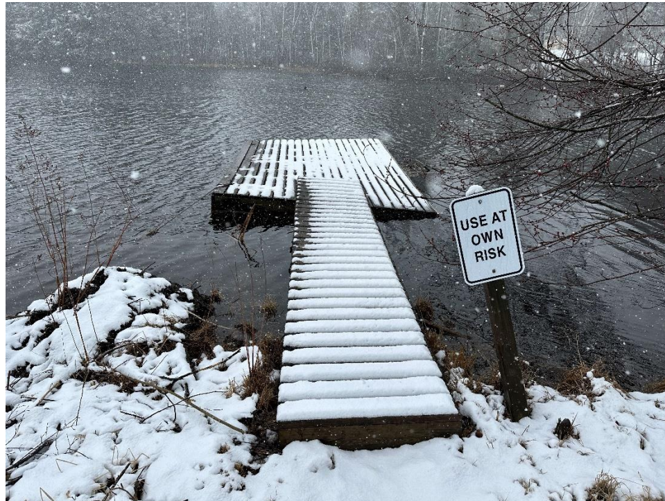
Photo 7 Typical Wood Dock
