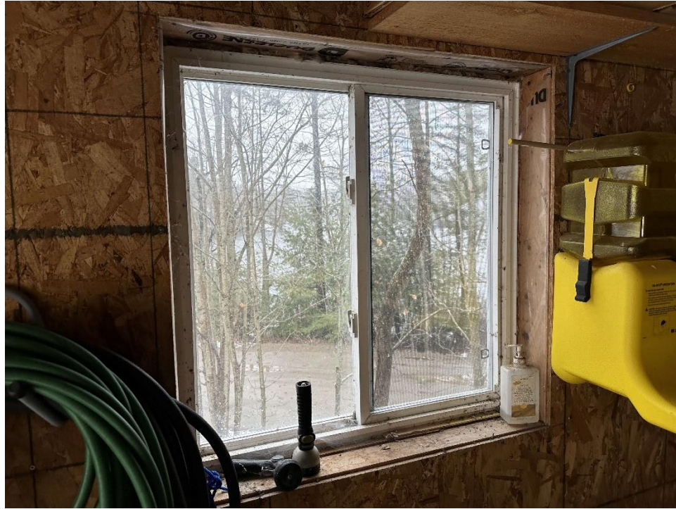
Photo 17 Operable window at Storage Building
