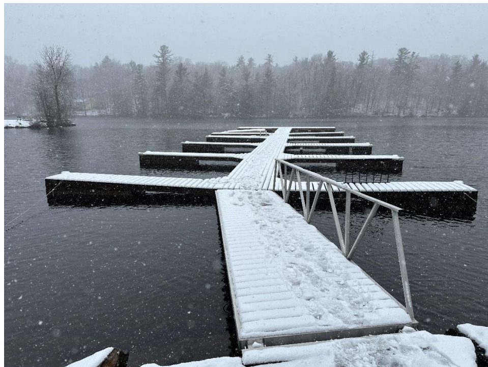
Photo 8 Typical Boat Docks (Wood and Aluminum Frame)
