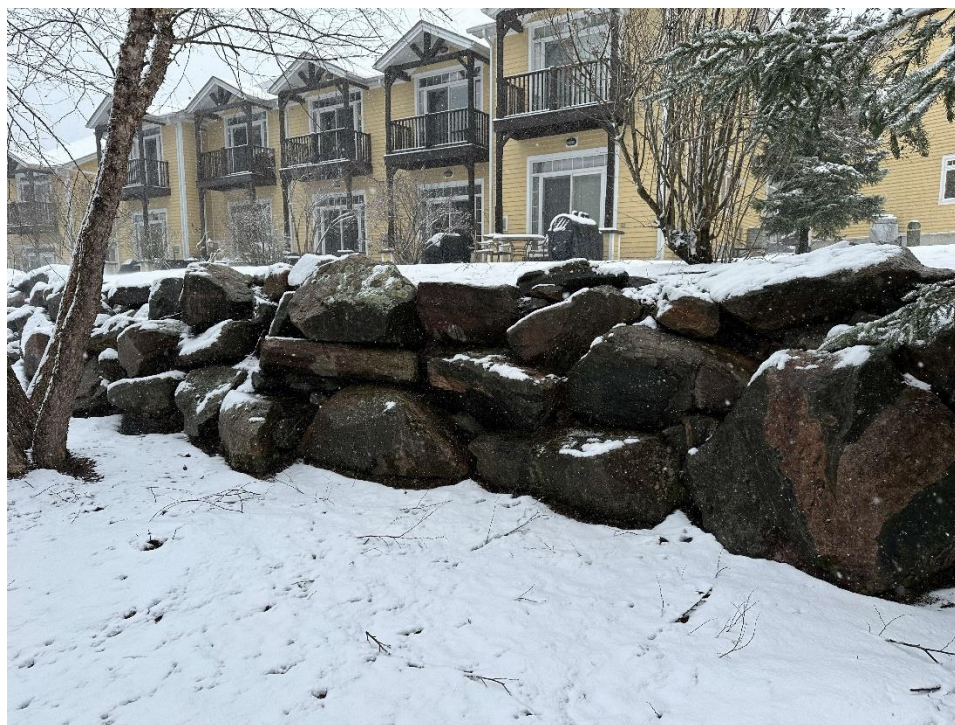
Photo 6 Typical Retaining Wall
