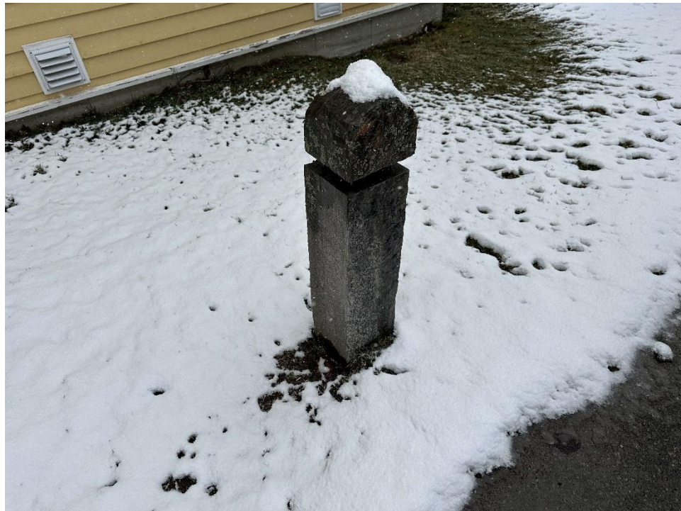
Photo 28 Concrete Bollard Light at Walkway
