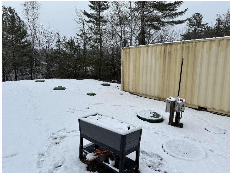
Photo 22 Septic Bed Overview (partial snow cover)
