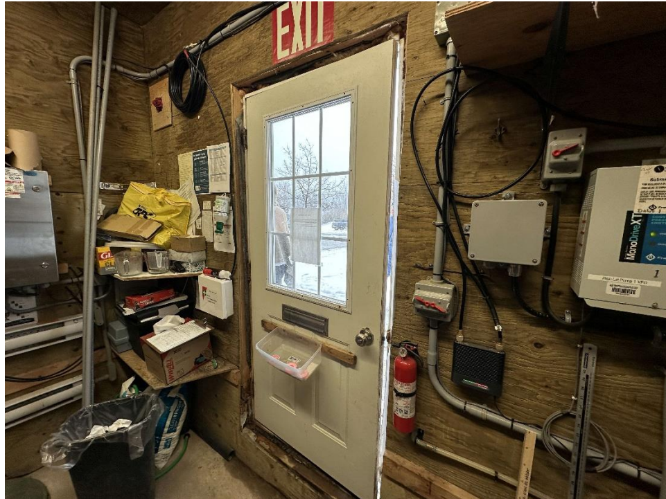
Photo 18 Painted Wood Door at Pump House
